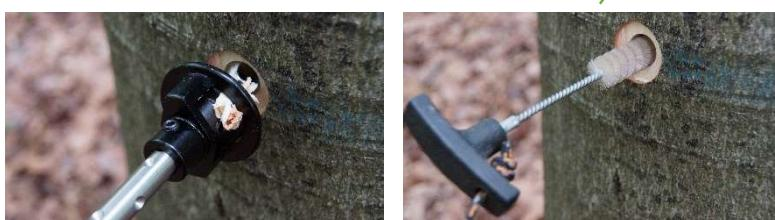
Create a stepped drilling, clean the borehole, disinfect the borehole, apply resin, screw in the platform bolt.
