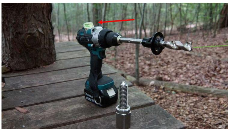
The creation of a step borehole is now carried out, taking into account the installation instructions for platform bolts ("Rev A // 06-06-2024") and with the use of a cordless screwdriver with a spirit level or a drilling jig.
