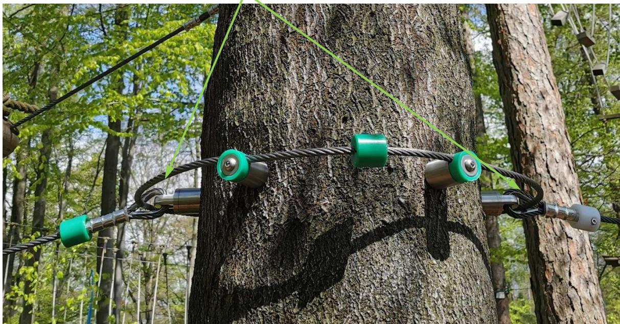
It must be ensured that the cable does not damage the tree's bark, e.g., by abrasion. If necessary, an abrasion protection (here rope carrier; see also 2.6) must be installed.
