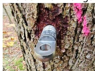
2.3.10 Screw in the middle load-bearing surface faces downward. The tabs are screwed in horizontally.
